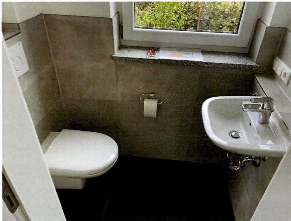
Foto 6: Blick in das EG-WC
